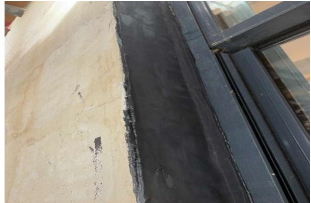
Ongoing EPDM Installation
