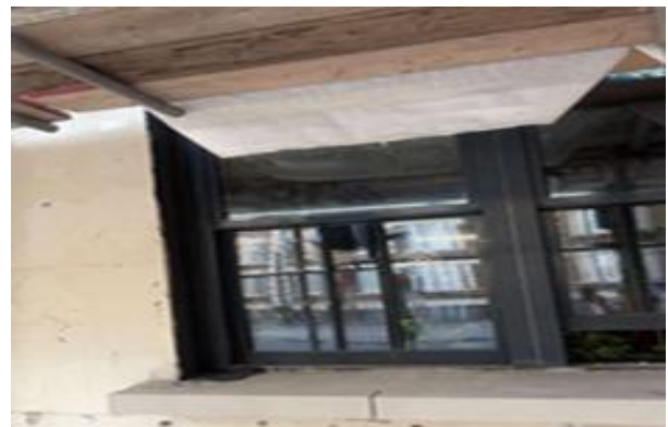
EPDM installation to the reveals
