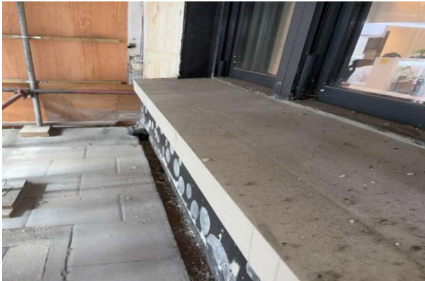
Ongoing Concrete repairs to Stonework
